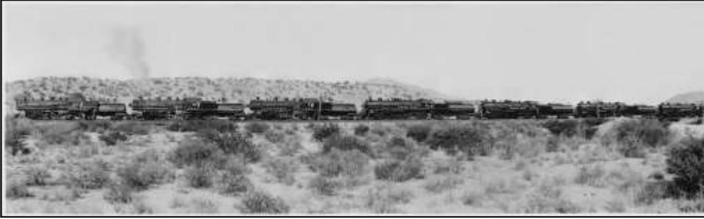
*Prosperity Special*—Twenty brand new 2-10-2 steam engines, part of a larger order of fifty for Marfa, Texas, June, 1922. The engines were being pulled by three 2-8-2 workhorse engines and trailed along on the publicity tour. This magnificent panoramic photo was produced by Duncan
