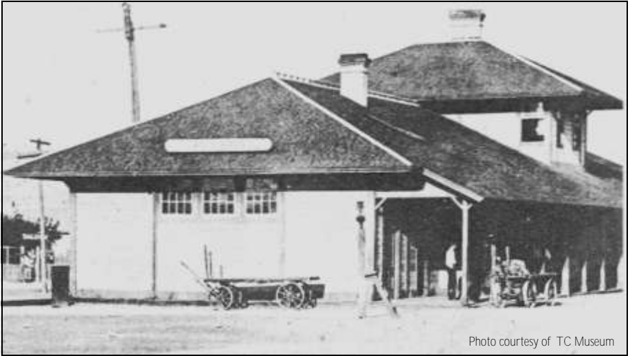
West end of the depot, ca 1909, before the 50' extension was added. The high windows let in light to a freight room, which had a wide door on the north side to receive freight for rail shipment.. The baggage wagons were used to move freight to and from the train. Massive wool and mohair shipments after the big sheep and goat operations were established necessitated the construction of a large freight house to the east of the depot.
