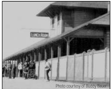
West end of the depot, ca 1909, before the 50' extension was added. The high windows let in light to a freight room, which had a wide door on the north side to receive freight for rail shipment.. The baggage wagons were used to move freight to and from the train. Massive wool and mohair shipments after the big sheep and goat operations were established necessitated the construction of a large freight house to the east of the depot.
