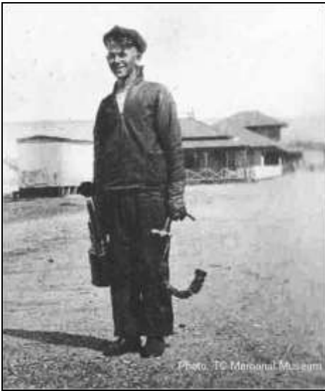
W. H. Lemons, Jr., railroad carknocker, with our house in the background, showing cross buck-style porch railings. Ca 1915
