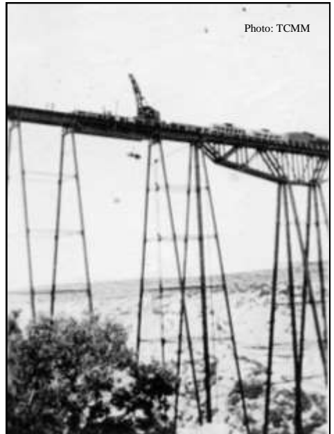
“Beefing up” the Pecos River Viaduct— maintenance on the world-class bridge.
