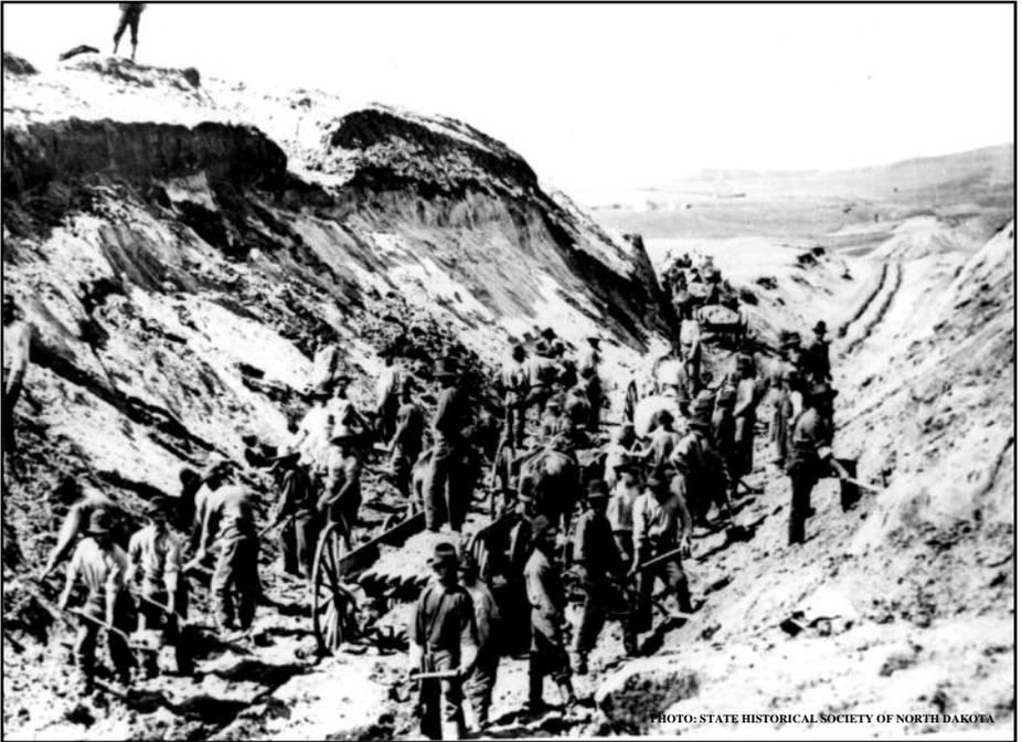
Much of the work done on the Southern Pacific route through Texas was done by manual labor. In the photo above, men working on the Northern Pacific make a road cut using hand tools, the same technology used on the SPRR.
