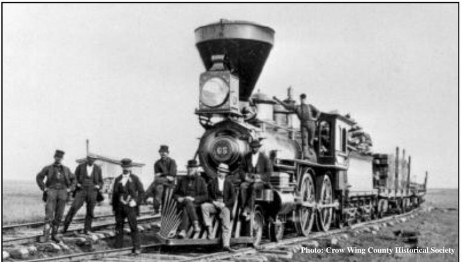
Not many construction photos are available for the building of the SPRR through Texas. This photo, taken on the NPRR, is a typical work train used in construction. The 4-4-0 engine was the workhorse of the world, with thousands of that wheel arrangement built for large railroads and small. The balloon-stack spark arrestor was a standard appliance in the dry west.
