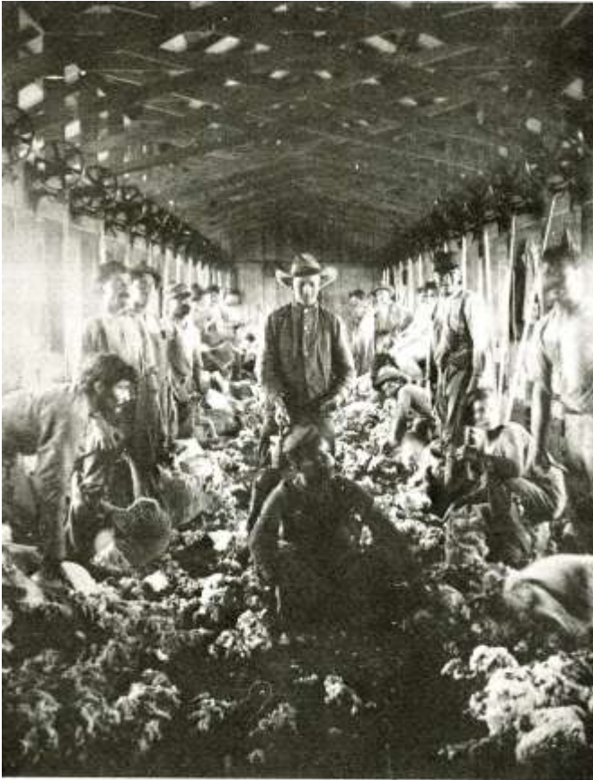
One of two shearing sheds on the ranch, forty machines and shearers kept a steady stream of animals moving through the process. A steam engine at the back kept the shearing machines running through drive shafts and pulleys located along the sides of the shed. This photo was made about 1915.
